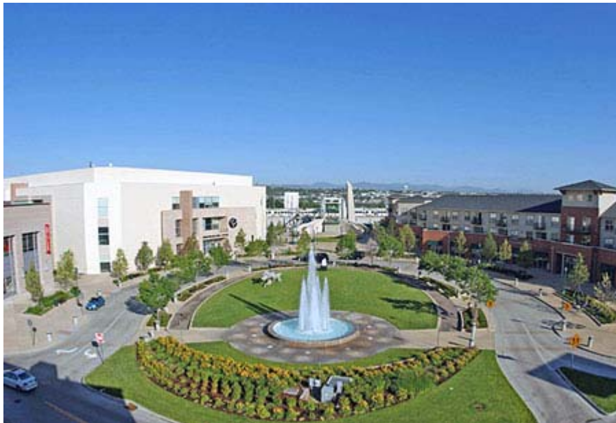
The Englewood Light Rail Station, along the RTD's Southwest Corridor Light Rail, has anchored local development since it opened in 2000. Credit: Courtesy RTD
